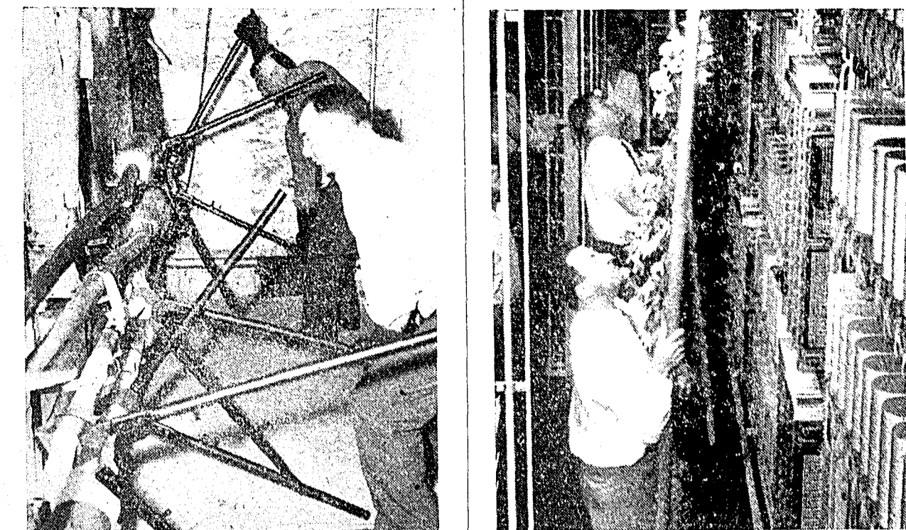
Telephone cable splicers are shown using large cutting tools to sever the cables in the basement of the old telephone building...
