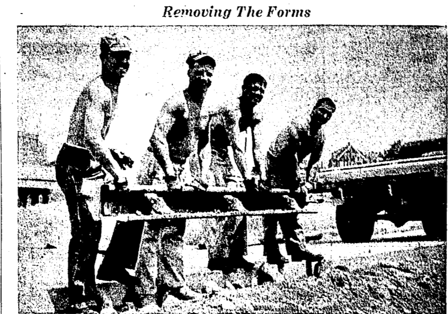
Workers remove the forms from pavement laid on the new exit from the relocated Route One roadway near Woodward Ave. Opening of part of the highway to one-way traffic is scheduled for tomorrow, to help relieve congestion on Main St. here. Second from the right is Walter Carpenter, of 132 Vista Dr.
