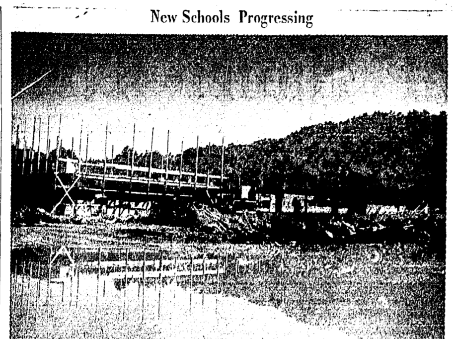
FOXTON SCHOOL. Reflected in a large pool left by recent rains, the new school being constructed in Foxton shows scaffolding around the all-purpose room which is nearing completion and the classrooms whose exteriors have already been dressed with brick veneer.
