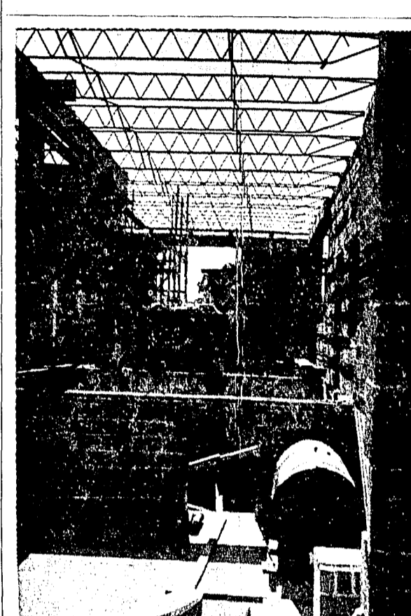
Roof jobs are shown in place over the boiler room at the new eleven-room school on Gerrish Ave. The jobs represent a landmark in the school construction here, since this is the first room on which a start has been made on the roof.
