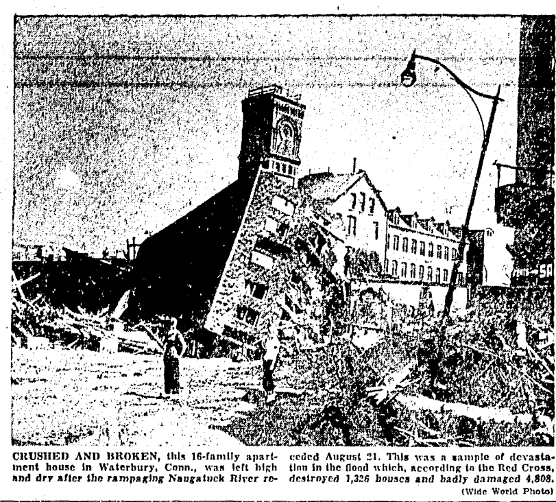
CRUSHED AND BROKEN. This 16-family apartment house in Waterbury, Conn., was left here in the flood which, according to the Red Cross, and dry after the rampaging Naugatuck River destroyed 1,325 houses and badly damaged 4,888.
