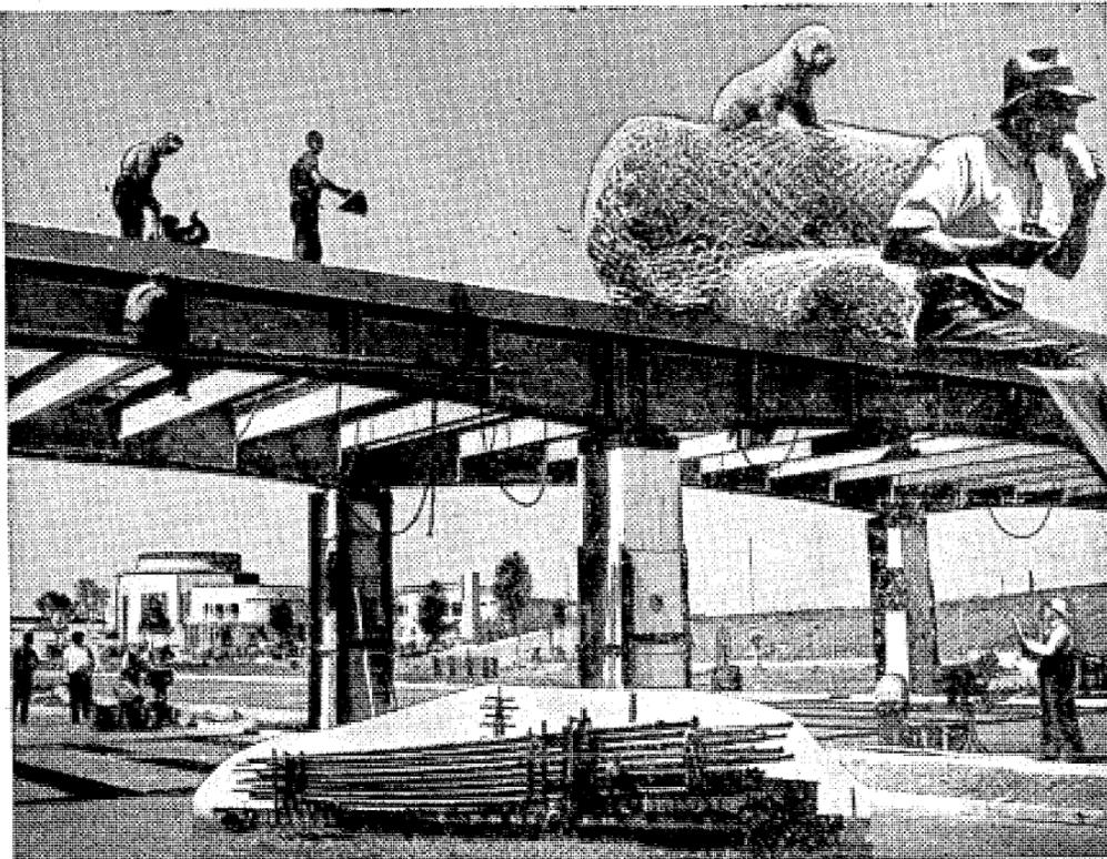
NEW YORK (Special).—There in the piers of the overpass is grey granite from Massachusetts capped by "pearl black" granite from Minnesota and supporting structural steel from Pennsylvania. Beyond are the posts for steel fencing made in Illinois, which will set off a building comprising \$900,000 worth of materials from many states that has been erected on Douglas fir pilings (see them arriving, insert) grown in Oregon and Washington and
