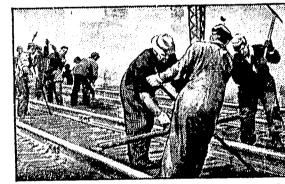
AUGUST... Miles of track relaid - re-ballasted almost 29,000 tons of rail installed for the year-in spite of shortages of men and materials. It is only by constant inspection and careful maintenance, that our right-of-way is able to stand up under the strair, and stress of wartime traffic.
