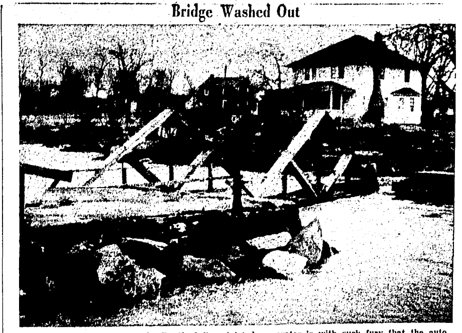
Bridge Washed Out Storm waves pounding into the Bradford Cove inlet drove water in with such fury that the auto bridge spanning the stream and connecting with the property of the Bartlett family was washed off its abutments.
